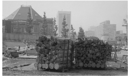
The recovered pine pylons at the redevelopment site of the Marunouchi Building.
